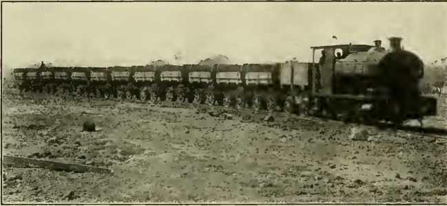
FIG. 1. CONSTRUCTION TRAIN ON BOMBAY DEVELOPMENT FITTED WITH M. C. B. COUPLERS
